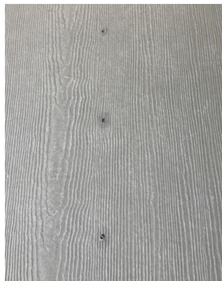
FIGURE 8. Water absorption at fastener penetrations.
